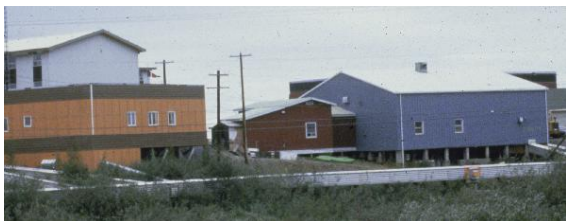
Buildings on Stilts in Tuktoyaktuk, NWT; Designed to Dissipate Heat and Avoid Permafrost Degradation
