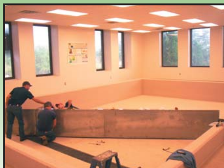
Assembly of custom-fabricated wave bulkhead.
