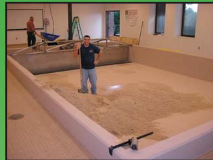
CE student shoveling the beach sand into the basin.
