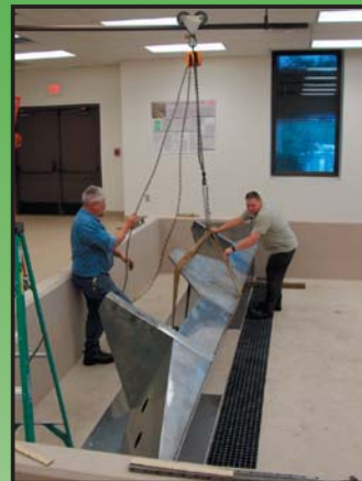
USA staff installing the wave bulkhead.
