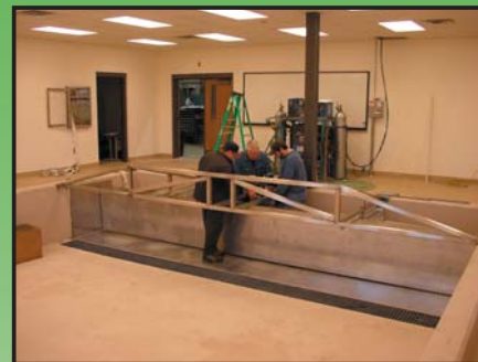
Installing the wave generator piston on the support frame.
