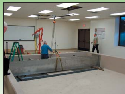
USA staff installing the wave bulkhead.
