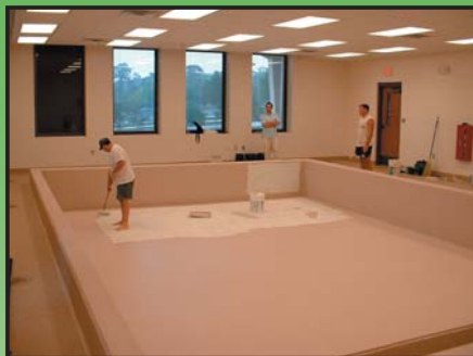
USA Civil Engineering (CE) students sealing the wave basin.
