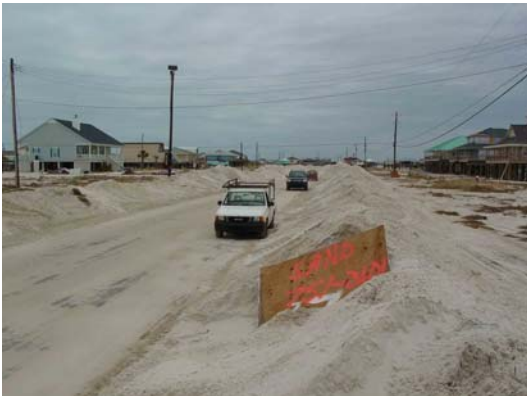
Photograph B. Bienville Blvd. was buried in sand during Ivan but the pavement was intact. Thus, the road was open immediately after sand removal. This intentional strategy, low elevation road construction, appears to have been successful at reducing pavement damages.
