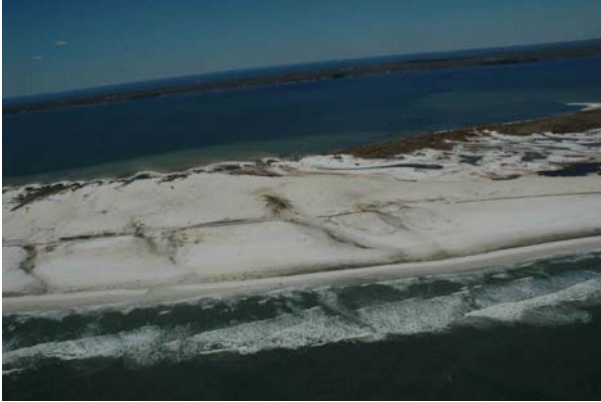
Photograph R. Damage to a portion of FL 399 in Gulf Islands National Seashore that had been relocated north to prevent such damage in 1996.
