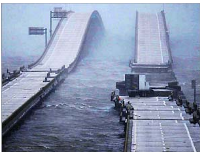
Photograph M. Interstate 10 bridge collapse into the Escambia Bay arm of Pensacola Bay (AP photo from web). This damage was from waves hitting the bridge decks due to the storm surge.
