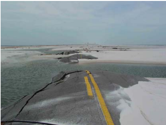
Photograph J. Pavement damage to Ft. Pickens Road in Gulf Islands National Seashore
