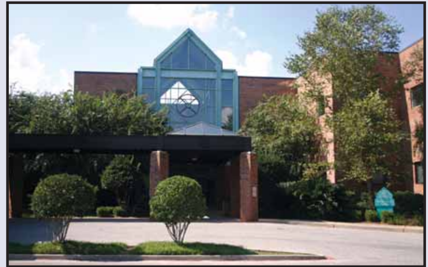
USA Technology & Research Park, Building III
