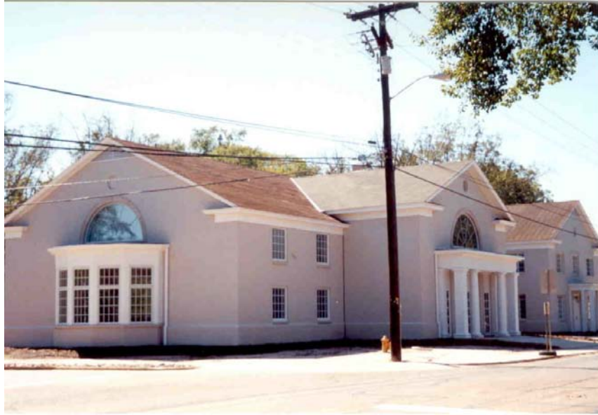
Completed Social Work Building
