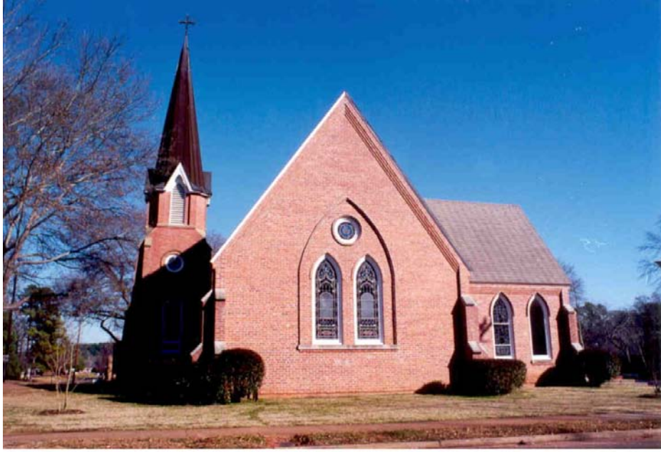
Social Work Building Before Remodeling
