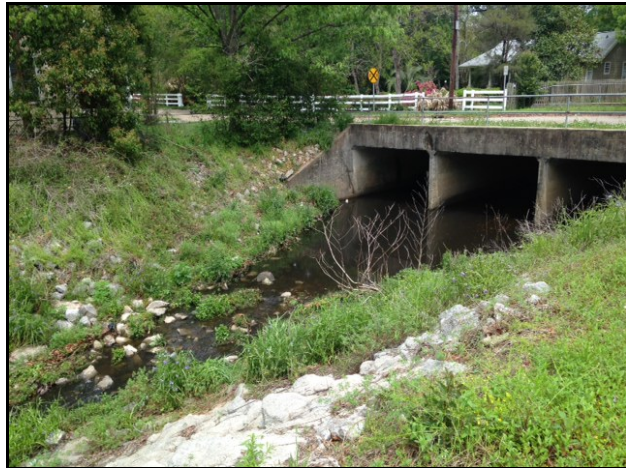
Figure 3. Transition from concrete to riprap channel
